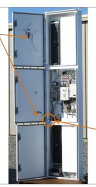
There is a little "gutter" above each door opening that holds water and may allow it to seep into the cabinet. Check that installer cut a slot in the side of the door "gutter" to let the water drain out.
